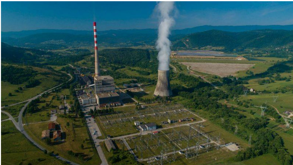
Fig. 2. Pljevlja thermal power plant
