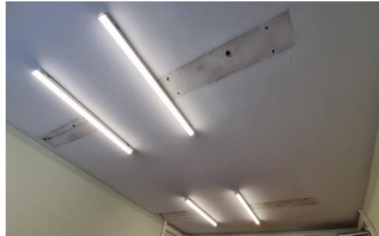
Fig. 14. New LED lighting immediately after installation
